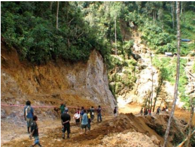
Road cut across spur with part of artisanal mining area in background.
